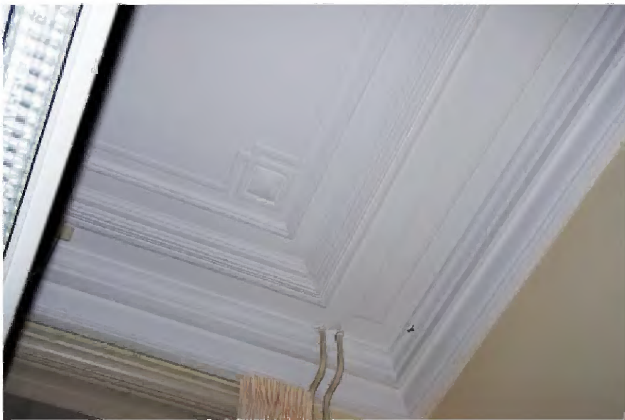
TK-B-78 Detail stucwerkplafond in B.01.0.02 circa 1900.
