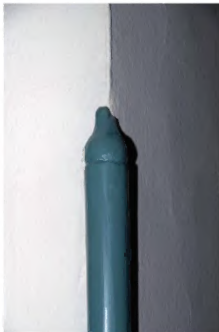
TK-B-105 Detail houten stoothoekkraal.
